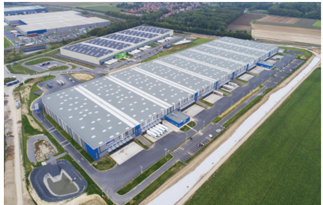
Lauwin-Planque Logistics Centre
