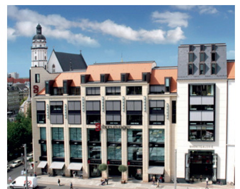
Marktgalerie, Leipzig, Germany, office, residential and commercial building
