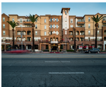
Tuscany Apartments, Los Angeles, California/USA, residential and commercial building
