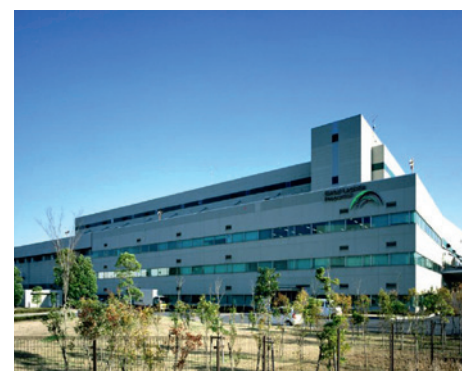
Narita, Chiba, Japan, storage/logistics building
