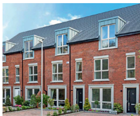
Cedarview, Santry, Ireland, residential building
