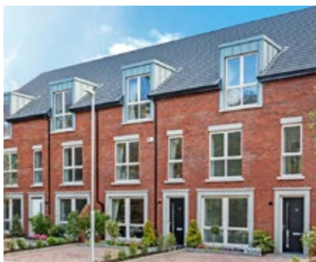
Cedarview, Santry, Ireland, residential building
