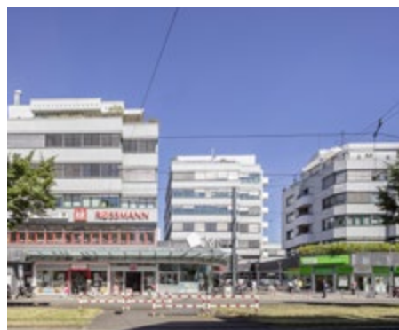
Münster Center, Düsseldorf, Germany, office, commercial and residential building
